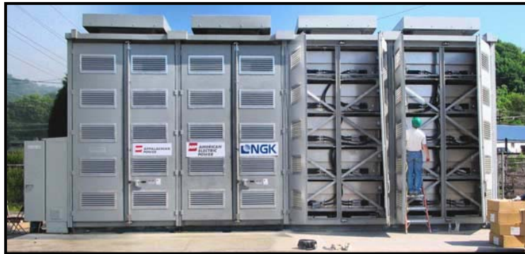
1.2 MW Sodium-Sulfur Flow Battery, Charleston, WV
