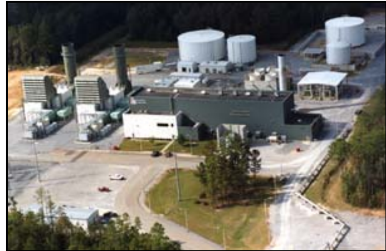
110 MW Compressed Air Energy Storage Facility, McIntosh, AL
